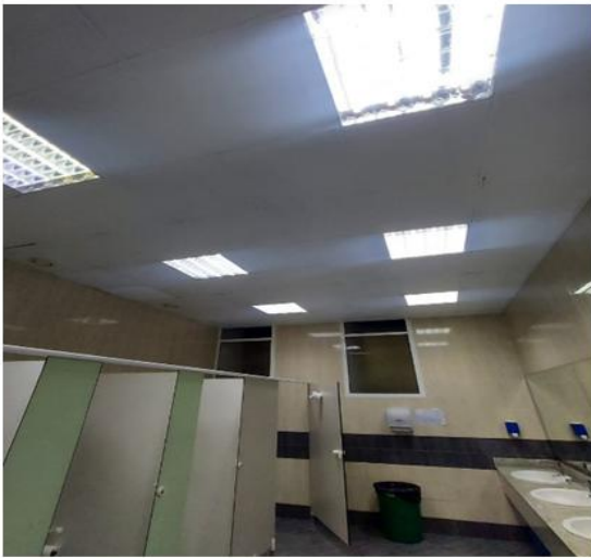
Fig 2 Washroom in J1
