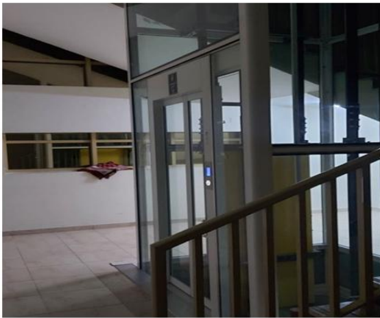
Fig 3 Corridor light in J2
